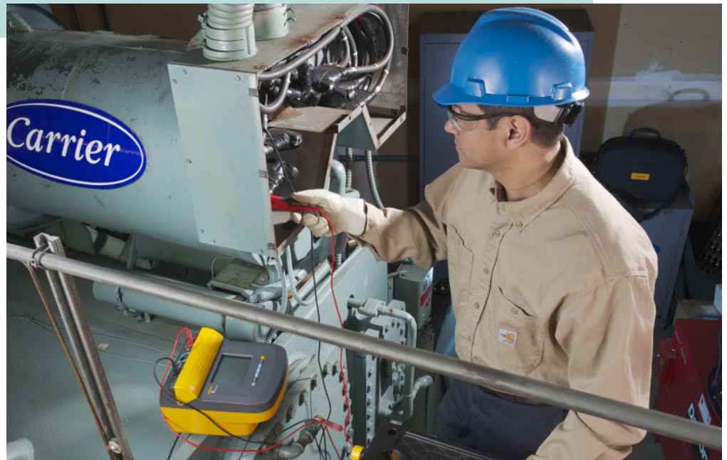
You can use a thermal imager, such as this Fluke Ti105, to check many parts of a boiler system.
